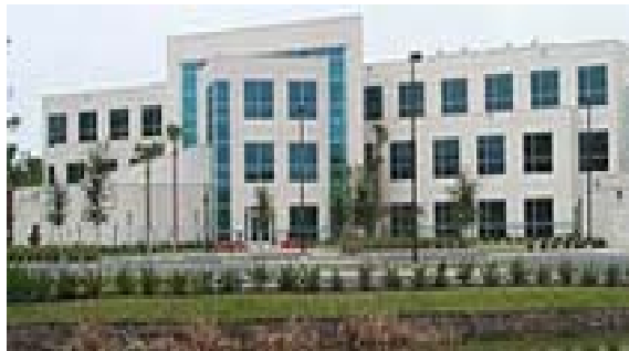
The National Center for Forensic Science Building
